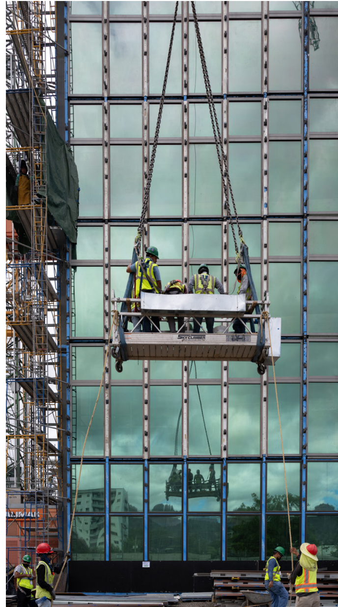
Images of site construction & mock-ups
