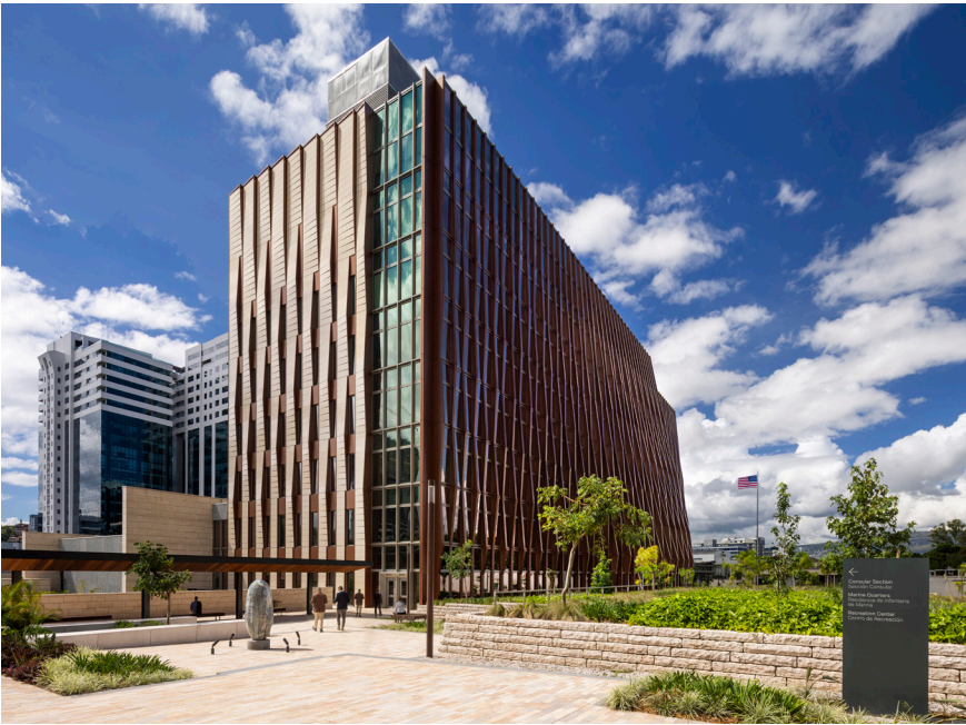
View of the Chancery from the CCAC entry court
