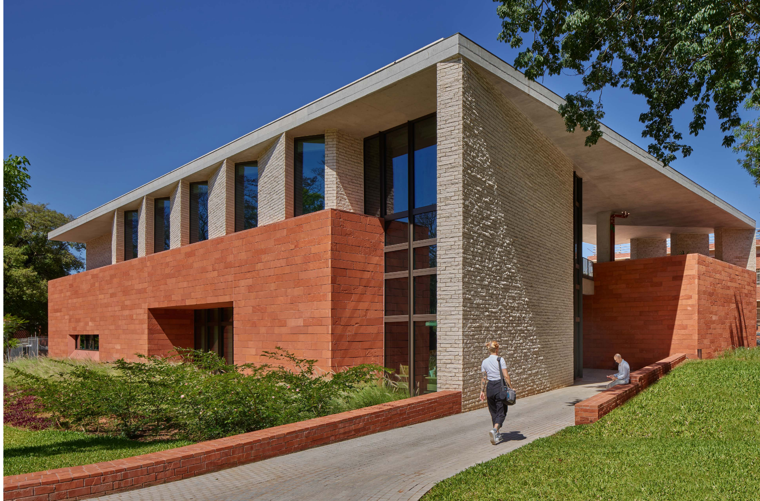
Passive control of sun and glare is a key driver in the design of the massing and how the materials are expressed.
